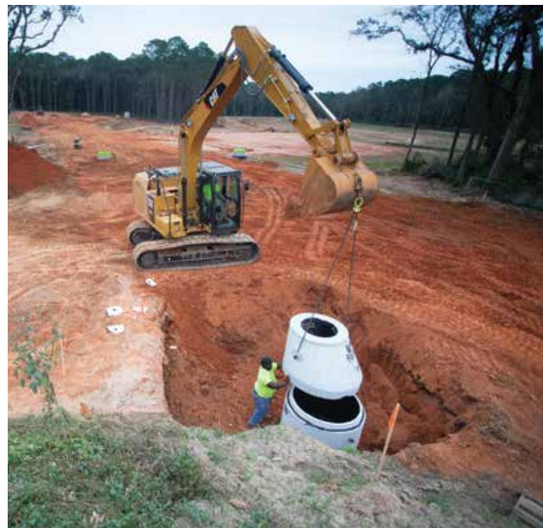
Top: A rendering shows the proposed free-standing emergency department, which is under construction on Hillcrest Road in west Mobile. Above: The construction crew works on preparing the site for the free-standing emergency department.
